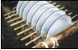
Plate rack detail using bamboo cane and elastic bands as well as traditional sisal lashings for main structure
