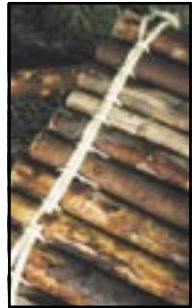
Alternative table top construction using logs.
